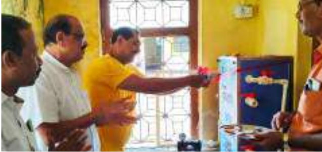
Water Filter Installation Palghar, Maharashtra
