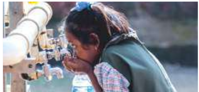
Water Filter Installation Palghar, Maharashtra
